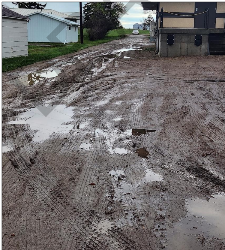
Figure 7: Ponding in Alley Behind Hospital, May 2024
