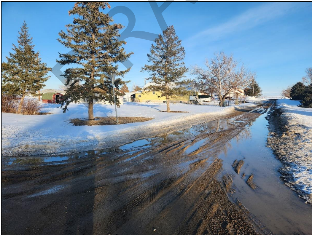
Figure 5: Ponding on McNamara Road, March 2023
