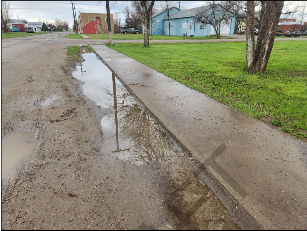
Figure 4: Ponding on 2 nd St, Date Unknown
