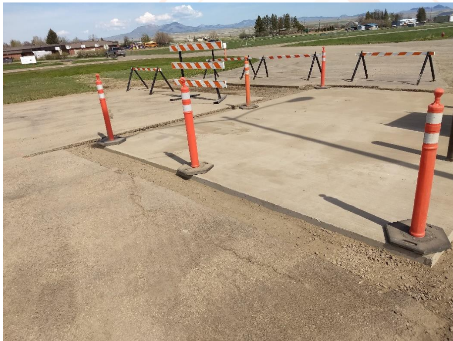
Concrete pad prepped for asphalt patching
