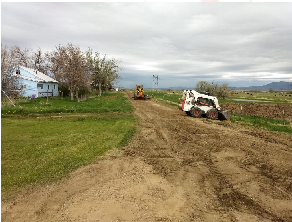
5 th Street finishing grading
