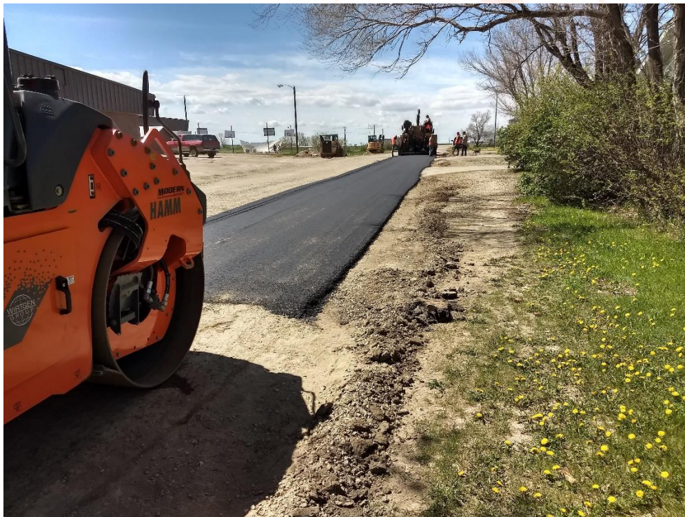
Roller compacting asphalt on 3 rd next to Elementary school
