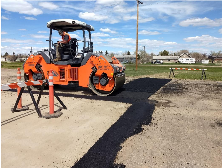
Roller compacting asphalt on 3 rd next to Elementary school
