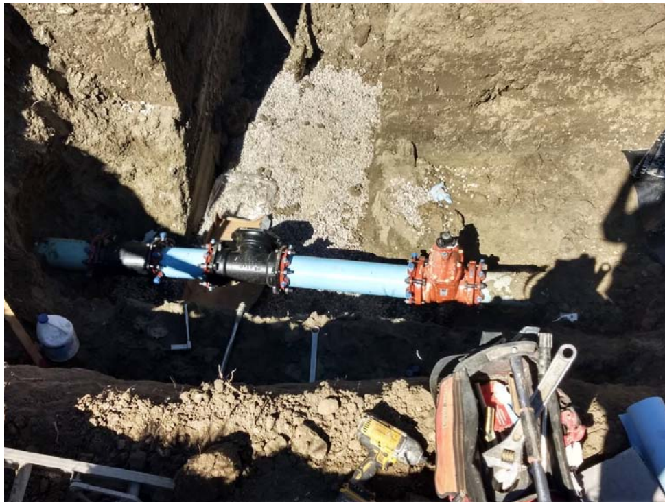
Installing new 6" tee and gate valve
