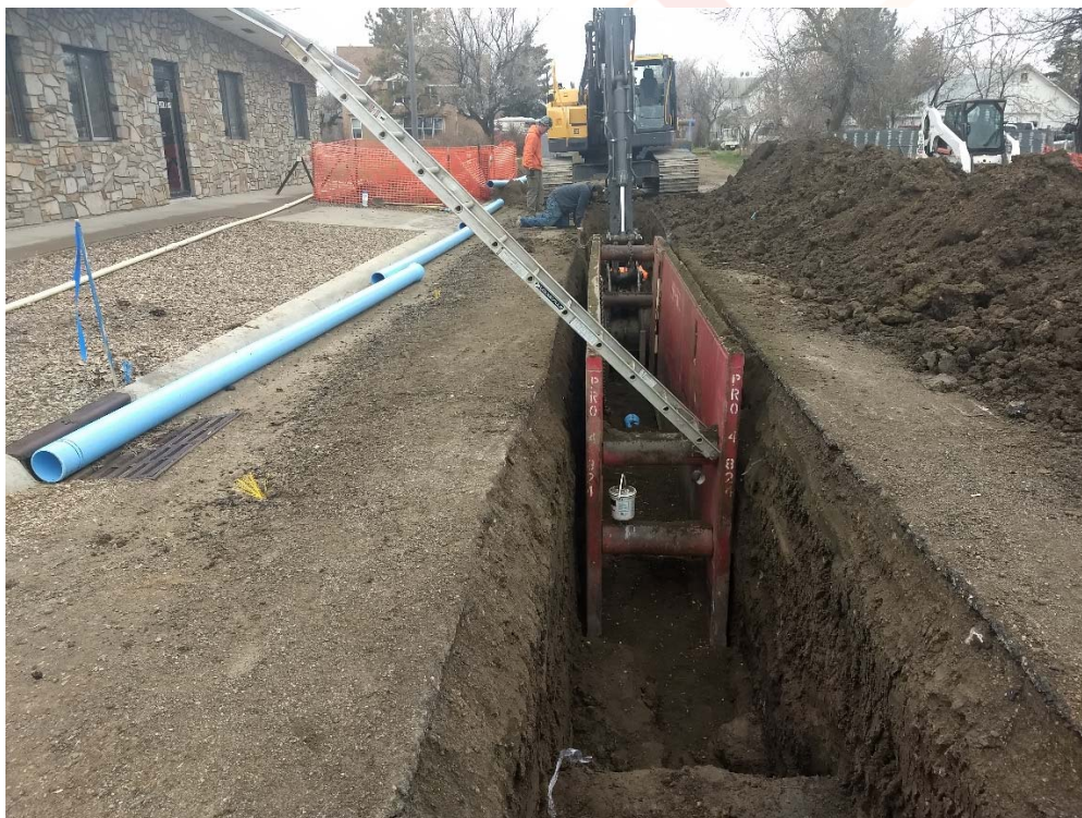
Installing 6" watermain along 1 st Street
