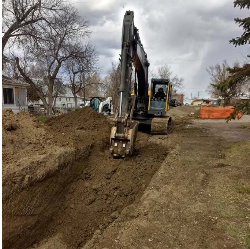
Backfilling and compacting on 1 st Street
